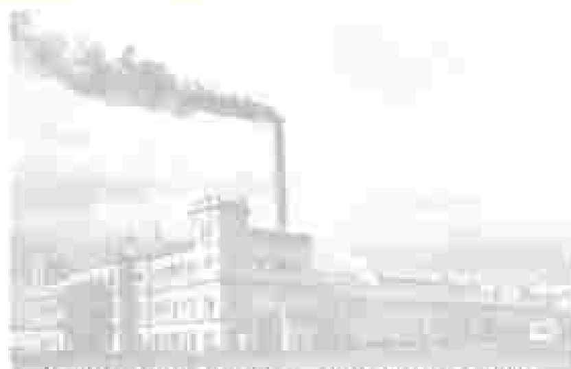
20 Kwatt BHU powerhouse (established in 1921)
